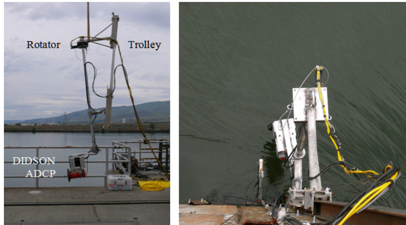
Figure 2.6. Photographs of a Trolley/Rotator Package for Deploying the DIDSON and ADCP (left) and the Loaded Trolley Being Lowered Down a 4-by-4-in. Box Beam at The Dalles Dam (right).
