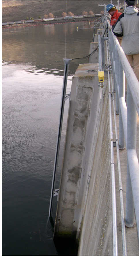
Figure 2.2. Pipe with Funnel for Acoustic Telemetry Trolley and Hydrophone Attached to a Powerhouse Pier-Nose at John Day Dam.
